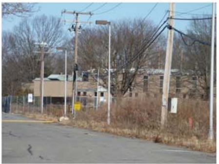
Vacant industrial site (13/1.02; Wyckoff Mills LLC).
