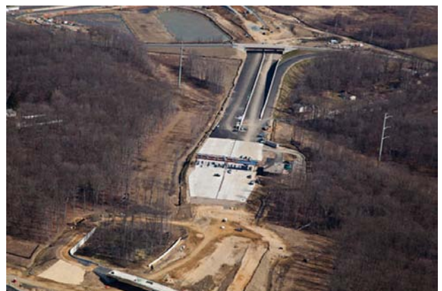
3/17/12 NJTA progress view of new Toll Plaza.
