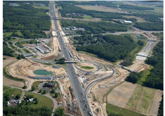
6/8/12 NJTA progress view of Interchange 8.
