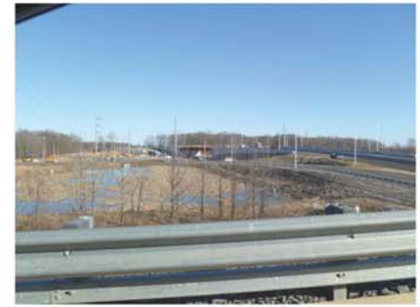
Detention basin between Milford Road and Rt. 133.
