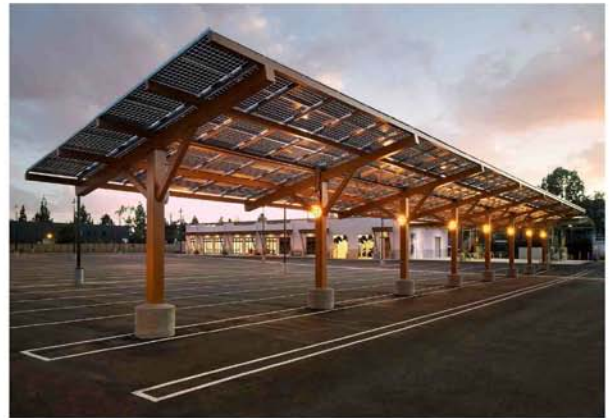
SOLAR PARKING LOT CANOPY
