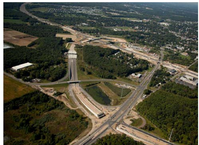
9/14/12 NJTA progress view of Interchange 8.
